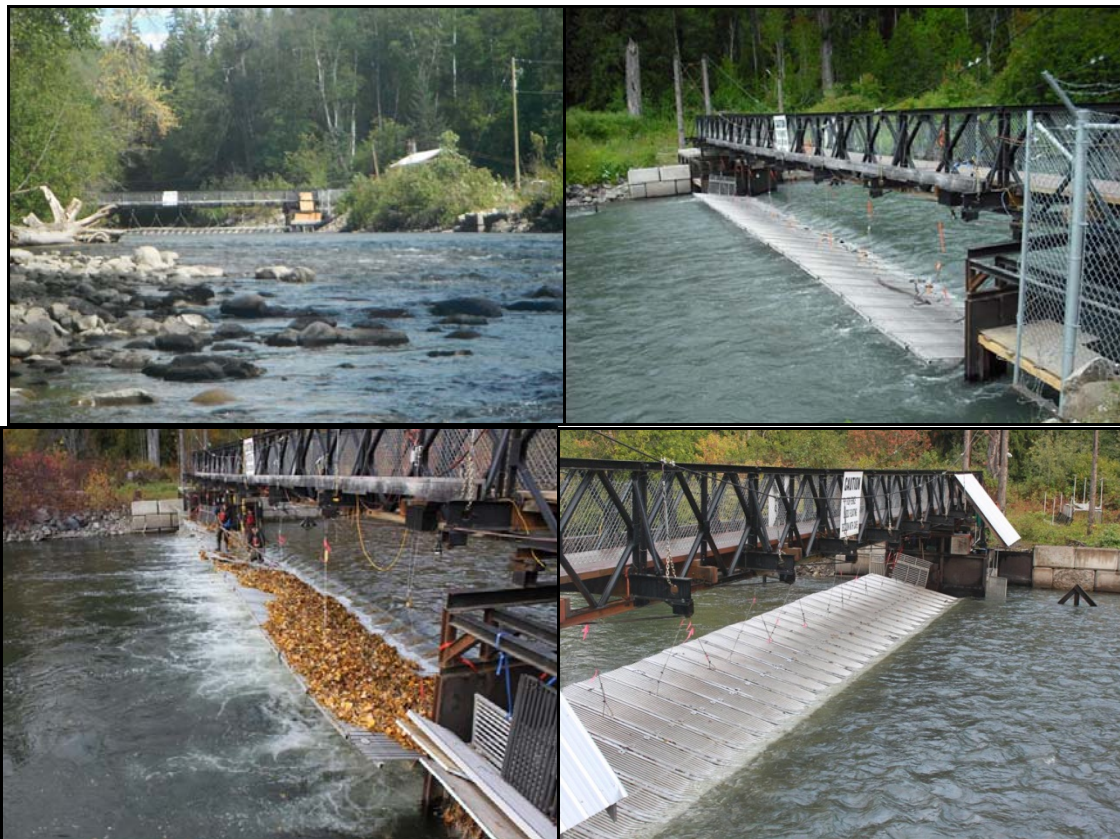
Figure 2: Photo series of the general KSEF structure including fence panels, right and left bank counting stations, overhead walkway, and winch cables suspended from the walkway that raise and lower fence panels according to flow rate and debris build-up.
