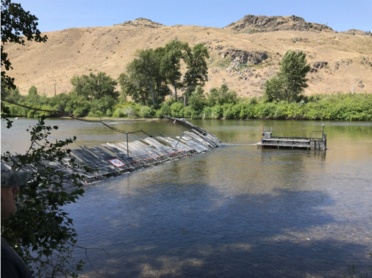
Figure 15. The CJH M&E weir on the Okanagan River downstream of Omak, Washington.
